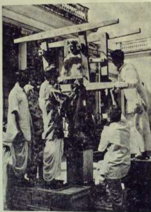
Hoisting of a Marble Stone
